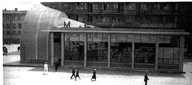
29. N. A. Ladovskii, the entrance pavilion to Krasnye Vorota metro station, side, 1935. MA, coll. 5, 6212.
